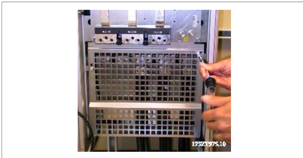
Illustration 3.39: Mounting of EMC shield.
