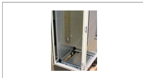
Illustration 4.27: Enclosure bottom cutout
